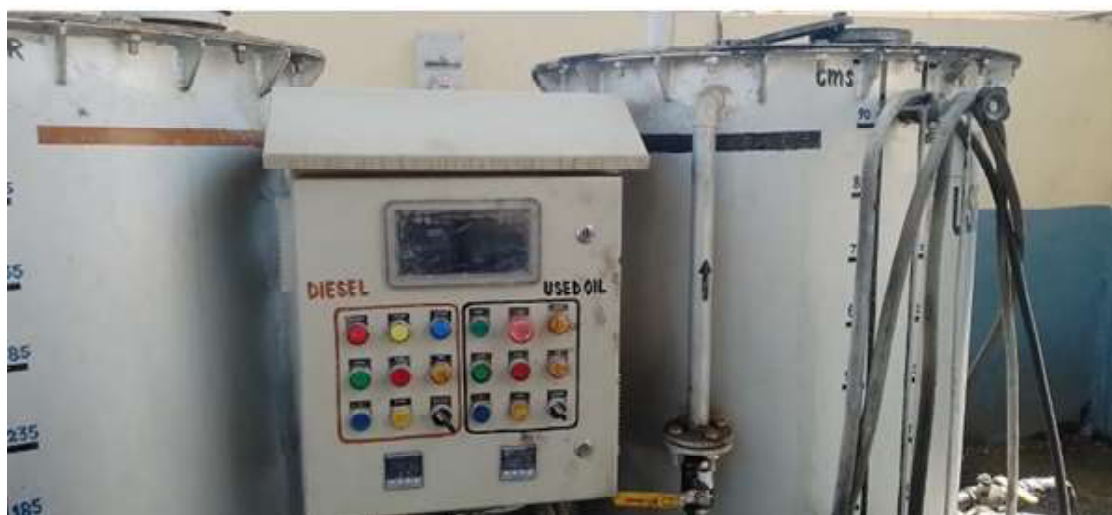
Figure 5 : Waste Oil Blending system
